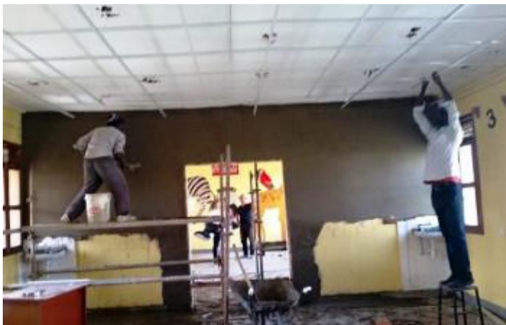
Workers refurbishing Ward 2
