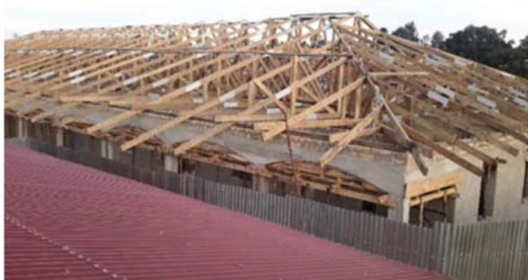
Raising the Roof.
