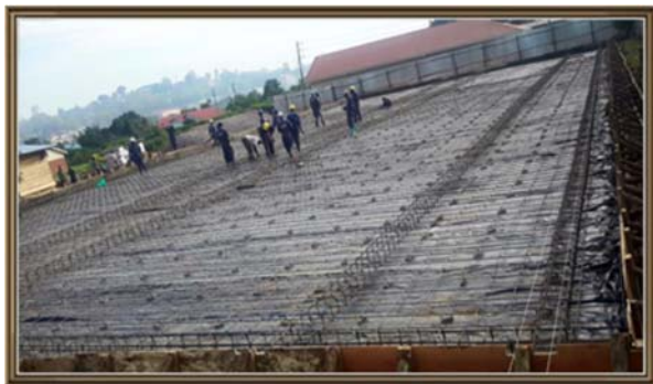
The Foundation is Laid.
